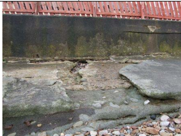
Cracking and erosion of concrete defences (Asset Ref No. 1221C901C0704C05)
