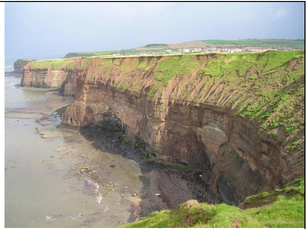
E59/4 looking towards Staithes from Redhouse Nab (Partly Active)
