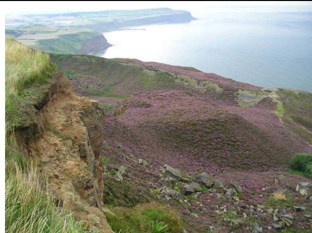
E58/5 looking west across the upper part of the disused alum quarries (Locally Active)
