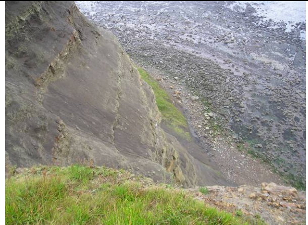
E54/2b erosion of lower cliff slopes (Totally Active)
