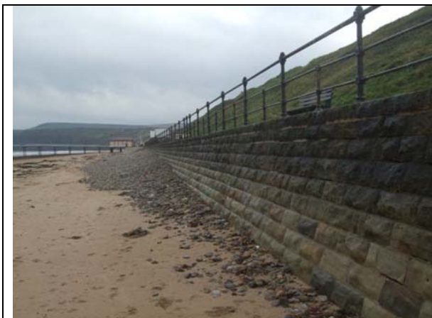
The sea wall at Saltburn (Asset Ref No's 1221C901C0703C02 to 1221C901C0704C06)
