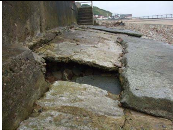
The mixed concrete and masonry defence (Asset Ref No. 1221C901C0704C05)
