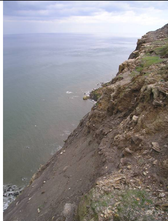
E58/4 (lower) looking east across the steep lower part of the disused alum quarries (Partly Active)
