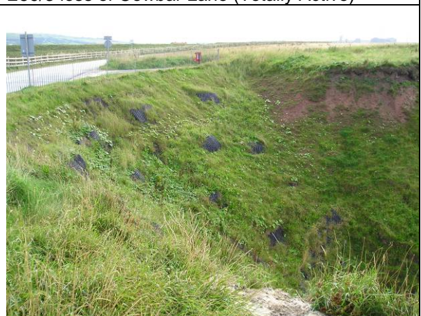
E59/1 flexible mesh facing near Cowbar (Partly Active)
